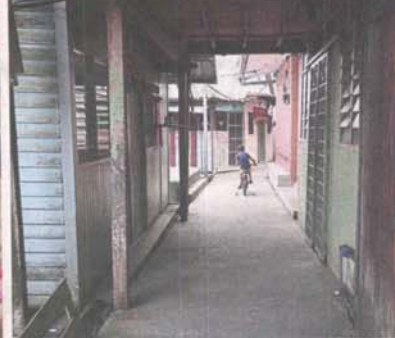
The state government plans to revitalise the village through the Breath New Life to Bagan Hailam programme.
